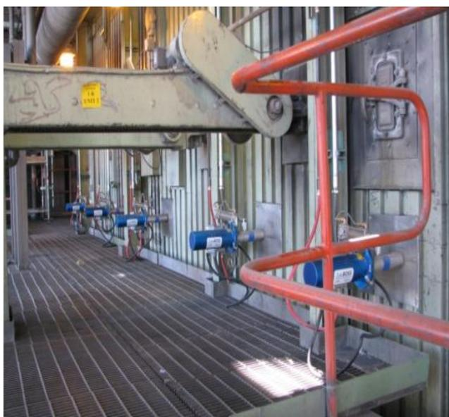
ZoloBOSS SensAlign heads mounted on the side of the furnace wall (above). The heads automatically realign as necessary to ensure optimum power transmission.
