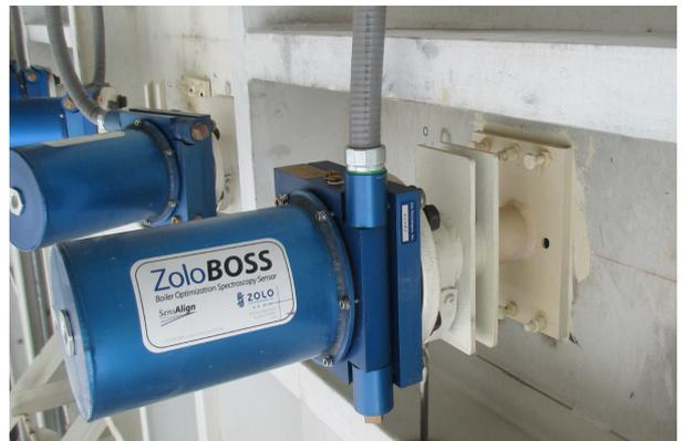
ZoloSCAN SensAlign heads mounted on the side of the furnace wall (above). The heads automatically realign as necessary to ensure optimum power transmission.
