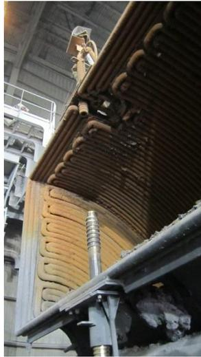
Figure 4. Original probe positions
